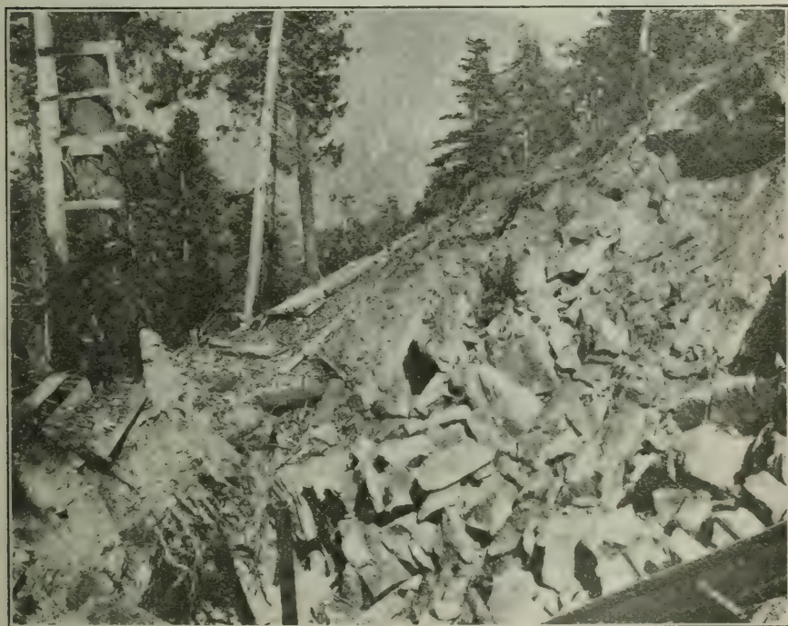
Photo No. 39. Edge of caved ground at surface of Little Castle Creek Mine, after extraction of the ore by caving system.
